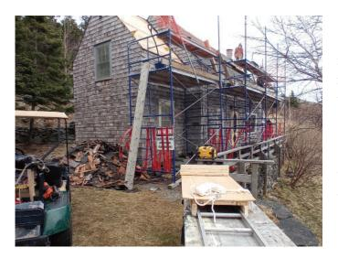
It is now nearing the end of April and Kent Cottage is getting ready for its new roof, roof number seven. With the help of Aaron and Byron Rodway of Rodway's Excavating and contractor, Anthony Noftle, the south side of the cottage is enmeshed in scaffolding, Jake's old cedar shake roof has been taken off and piled on the ground and a protective layer of Ice and Water Shield applied to the roof boards. Until we complete the wood shingling, this underlayment will keep out the water.
