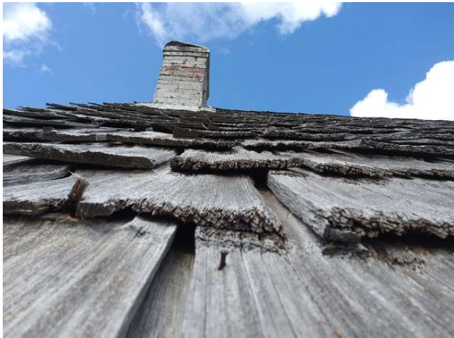
In 2022, the shingles are so brittle and eroded that they are literally breaking in two. Photo by Rex Passion.
