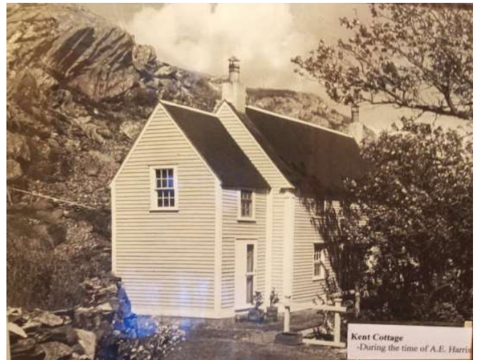
This photo by an unknown photographer shows Harris's brand new cedar shingle roof around 1927. The shingles were painted red.
